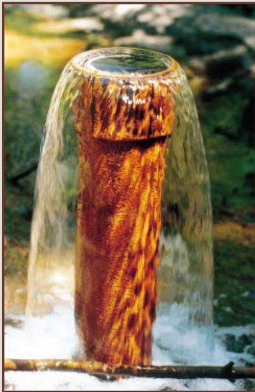
**Figure 5.** Depressurizing well flowing more than 100 gallons per minute near the MDA.
